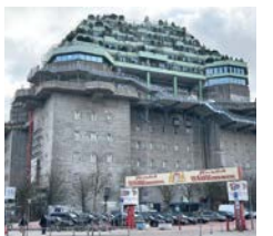
Medienbunker in Hamburg (Foto: proaudio.academy)
